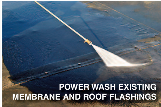
EPDM ROOF TO BE COATED
