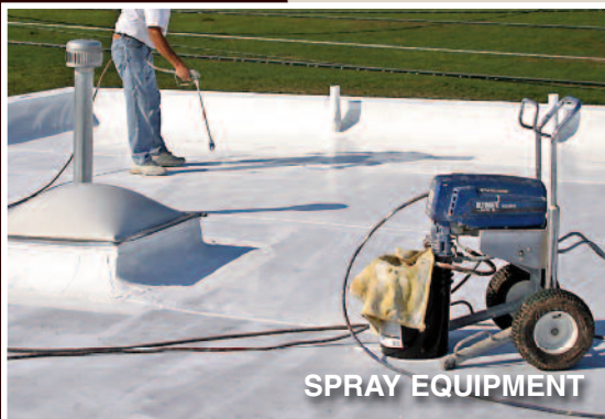
SPRAY APPLY SECOND COAT OF ROYAL EDGE RE-FLEX COATING
