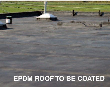
POWER WASH EXISTING MEMBRANE AND ROOF FLASHINGS
