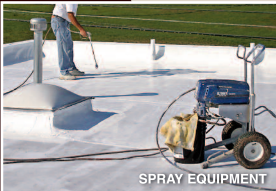
SPRAY SECOND COAT OF RE-FLEX COATING
