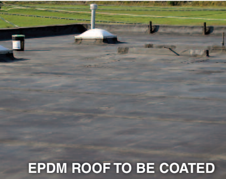
POWER WASH EXISTING MEMBRANE AND ROOF FLASHINGS
