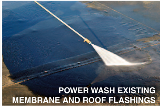
EPDM ROOF TO BE COATED
